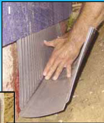
A TRENCH IS DUG IN THE EFFECTED AREA WHERE WE INSTALL OUR DOUBLE CURTAIN DRAIN™ PROTECTOR TO STOP DIRT FROM CLOGGING OUR WATER TREK AQUA ROUTE® CONDUIT.
