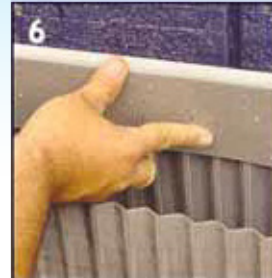
A SPECIAL "COVER PIECE" IS INSTALLED OVER THE TRENCH PROTECTOR STOPPING WATER FROM GETTING TO THE SILL PLATE.
