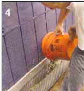
STONE IS BACKFILLED INTO THE CURTAIN DRAIN™ SYSTEM. GRAY IS THE STANDARD COLOR USED. WHITE OR OTHER COLORS CAN BE SUBSTITUTED UPON REQUEST.
