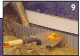
A SPECIAL "COVER PIECE" IS INSTALLED OVER THE TRENCH PROTECTOR STOPPING WATER FROM GETTING TO THE SILL PLATE.
