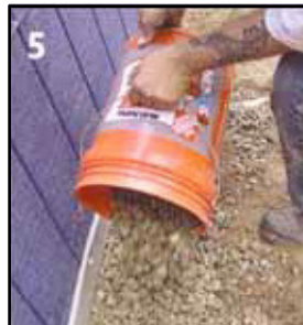
STONE IS BACKFILLED INTO THE CURTAIN DRAIN™ SYSTEM. GRAY IS THE STANDARD COLOR USED. WHITE OR OTHER COLORS CAN BE SUBSTITUTED UPON REQUEST.
